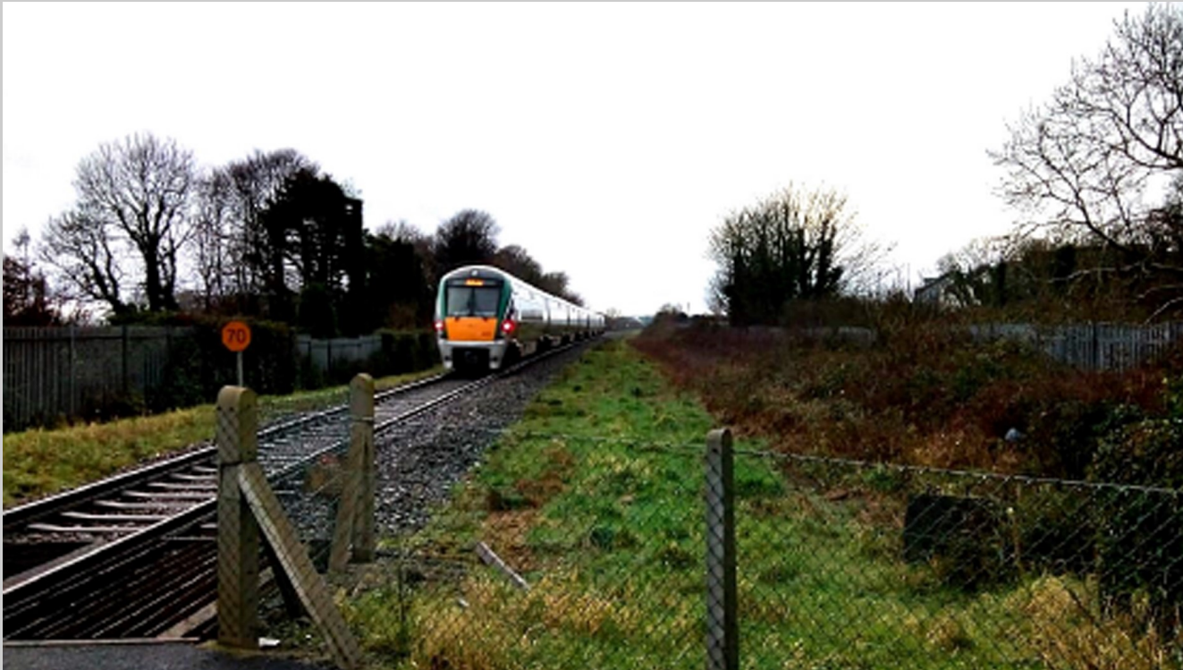
Murrough Level Crossing
